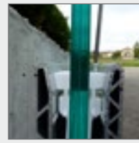
Simultaneously adjust vertical alignment and tighten clamp
