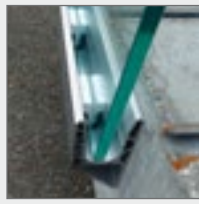
Install the glass
