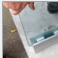
Install the glass
