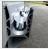
Install the U wedges
