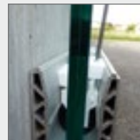
Simultaneously adjust vertical alignment and tighten clamp
