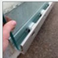
Install the glass
