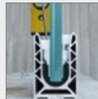
Simultaneously adjust vertical alignment and tighten clamp
