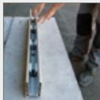
Install the U wedges
