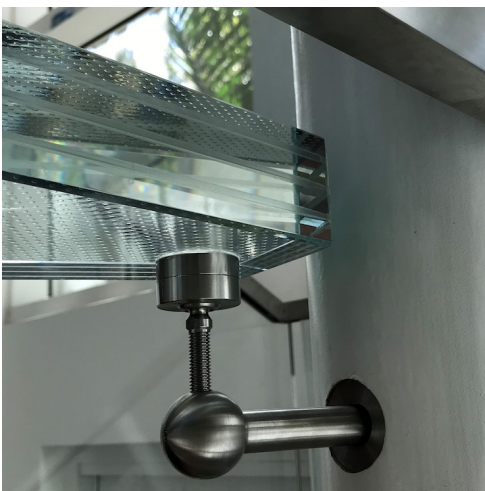
Custom Glass Stair Hardware with TSSA Fitting
