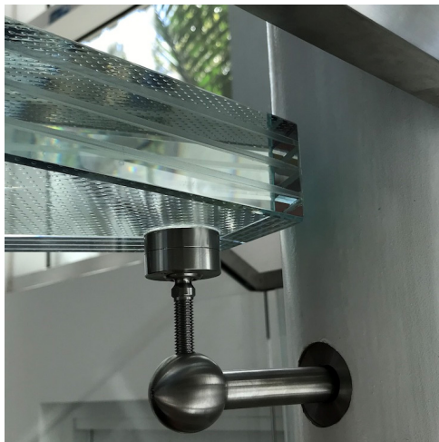
Custom Glass Stair Hardware with TSSA Fitting
