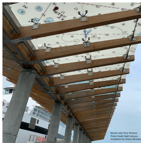
Custom Saddle Brackets on Wood Outriggers with S3100 & R1006 Fittings
