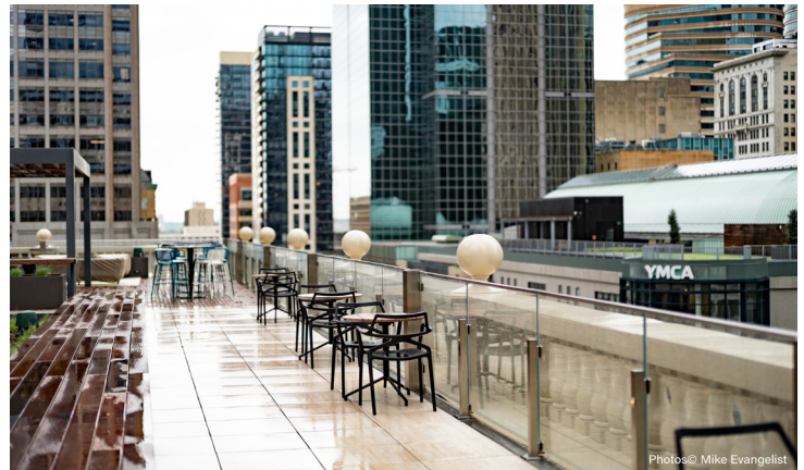
Custom Fabricated 6 x 6 and 2 x 2 Stainless Steel Posts with Welded Baseplates Fabricated, drafted & engineered by SADEV USA
